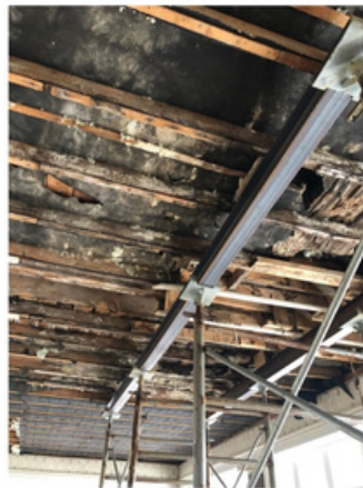
Details of damage to joists and supporting scaffolding.
