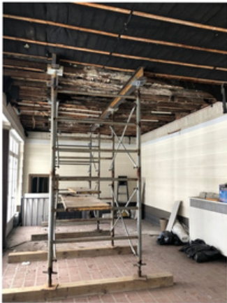
Interior view; doorway connecting to hallway located in lower left corner
